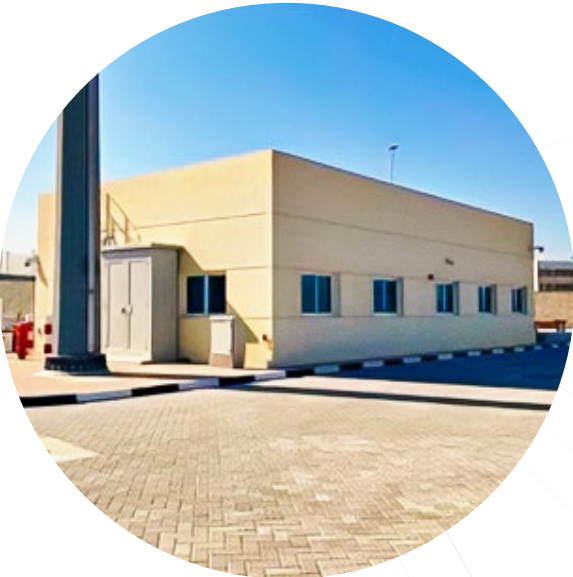
Satellite fuel station 2 ▶
